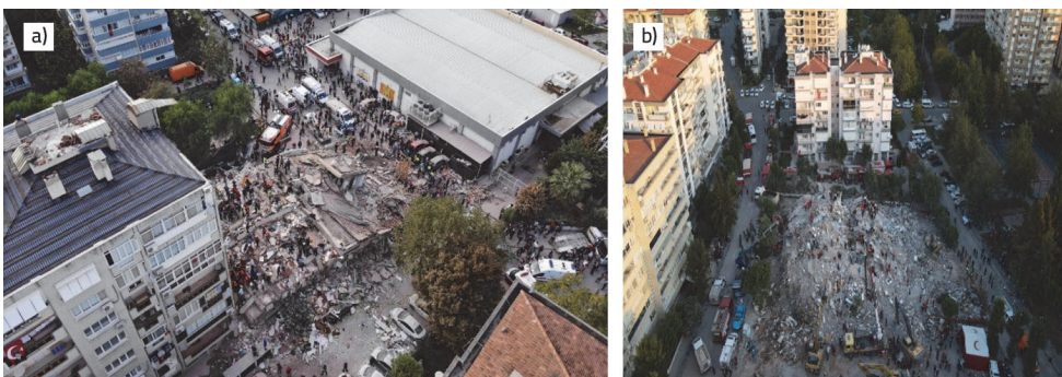
Figure 1. a); b) Failure of modern buildings during recent earthquakes
