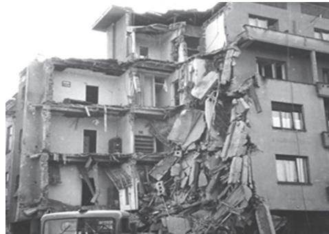
Figure 4. Partial failure of the masonry building, Banja Luka 1969
