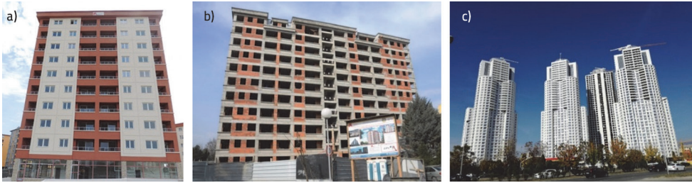
Figure 1. a) 9 story building; b) 10 story building under construction; c) 42 story buildings
