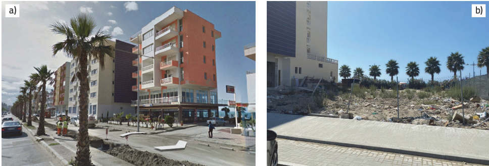
Figure 4. a) Building before demolition; b) The plot after demolition
