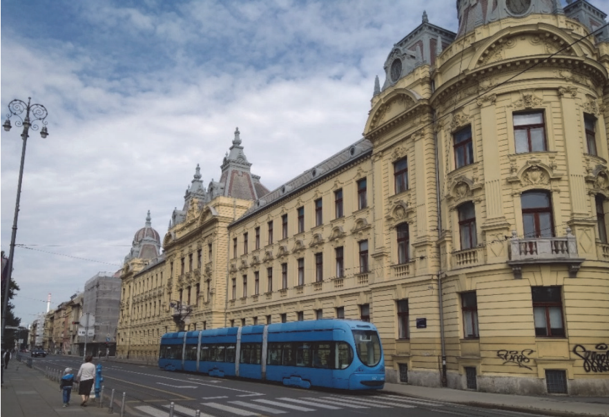
Figure 5. Tram passing in front of HŽ Infrastructure head-office building
