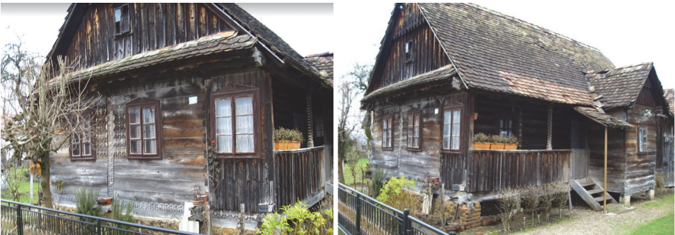
Figure 5. Wooden house in Mečenčani, on the fault of the December earthquake, without any damage. Wooden houses in the area suffered occasional plaster peeling, but generally no structural damages
