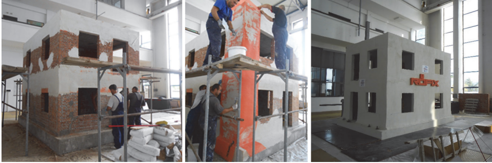
Figure 2. Retrofitting of the model using System RÖFIX SismaCalce
