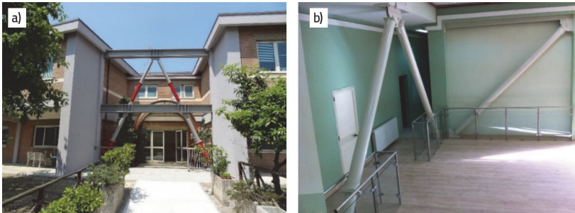
Figure 4. Buckling Restrained Axial Dampers (BRAD®) as installed in the Marsciano school in Perugia (a) and in the Consolino school in Vittoria, Italy. Source: [30]
