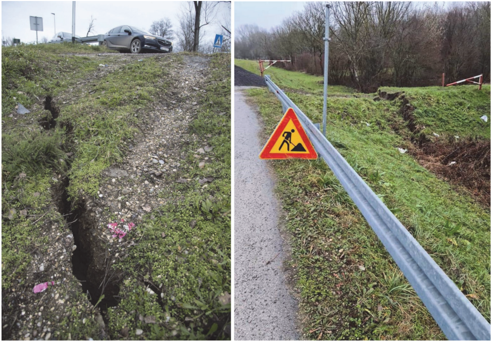
Figure 5. a) Surface fault crossing the Kupa riverbank at Brest Bridge, b) Surface fault rupture crossing the Sava riverbank at Palanjek (CREDIT: Public media).
