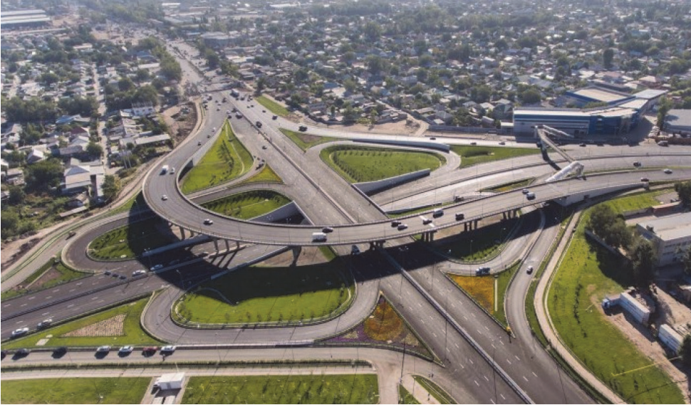
Figure 3. Aerial view of the Saina-Ryskulova bridge in Almaty (courtesy of Kazroadinnovation LLP)
