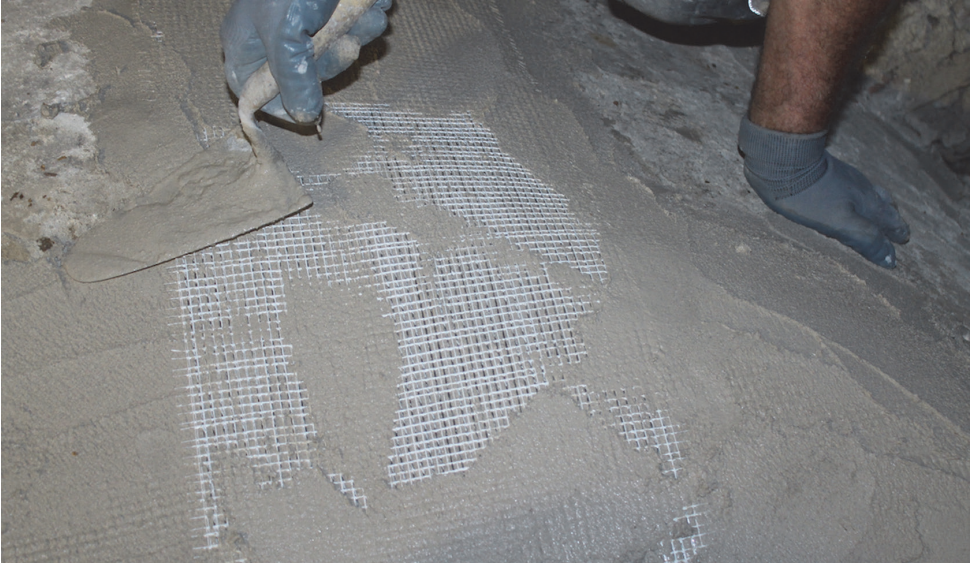
Figure 9. UHTSS steel net and lime mortar on the vault
