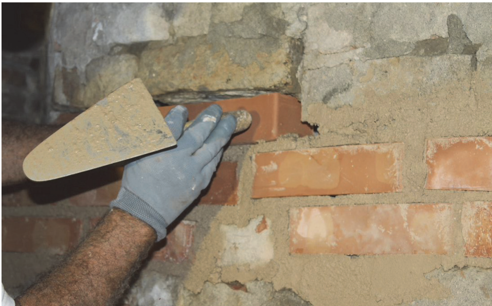
Figure 8. Rocca of Sissa cuci scuci with brick and lime mortar
