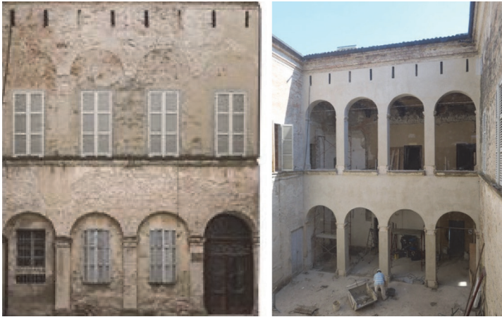
Figure 5. Rocca of Sissa, Inner prospect on the galleries, before (left) and after (right),
