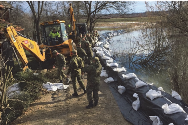
Figure 5. Reconstruction of the dyke
