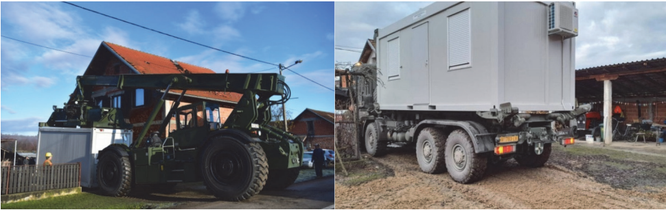
Figure 4. Installation of the container houses
