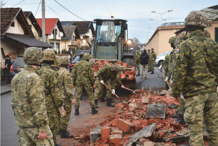
Figure 2. Reconstruction of roadways – manually
