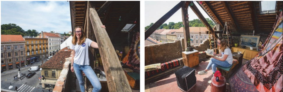
Figure 4. Zagreb, Ilica street, attic after the March 2020 earthquake, author Ivana Rakamarić source: https://www.24sata.hr/news/od-velike-rupe-u-zidu-napravila-terasu-imam-pogled-na-ilicu-693876
