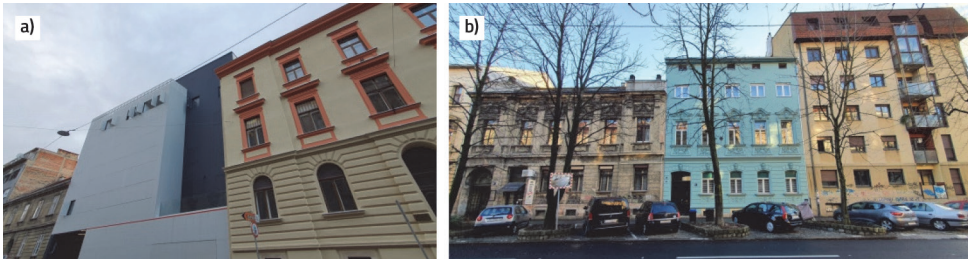
Figure 3. a) Kačićeva street 8, new building (author Matej Bender) adjacent to Kačićeva street 6, old building with a recently renovated façade - infill, “interpolation” b) Prilaz Gjüre Deželića 61, old building with a facade renovated according to conservation rules; building has two floors that were added throughout history
