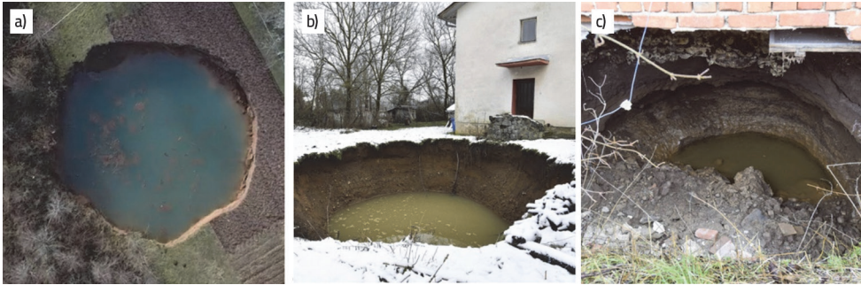
Figure 3. Holes in the ground as a result of the earthquake in the village of Mečenčani. a) Aerial view, b) Hole next to the house (source: Damir Krajac / Cropix), c) Hole under the house (source: Darko Tomas / Cropix)
