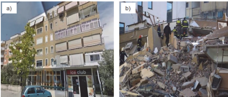
Figure 4. USAR search and rescue operations on six story reinforced concrete building in Durrës built in 1996: Before and after earthquake [10]
