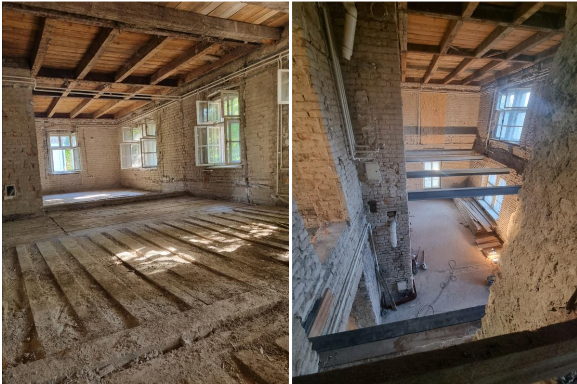
Figure 8. Plaster removal and preparations for strengthening
