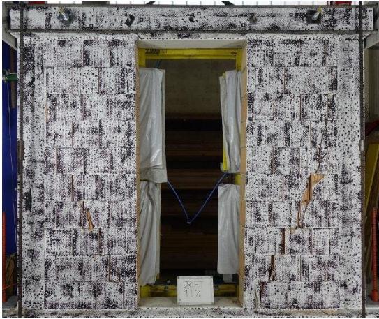
Figure 5. Damage to masonry infill at 1.1 % of in-plane drift
