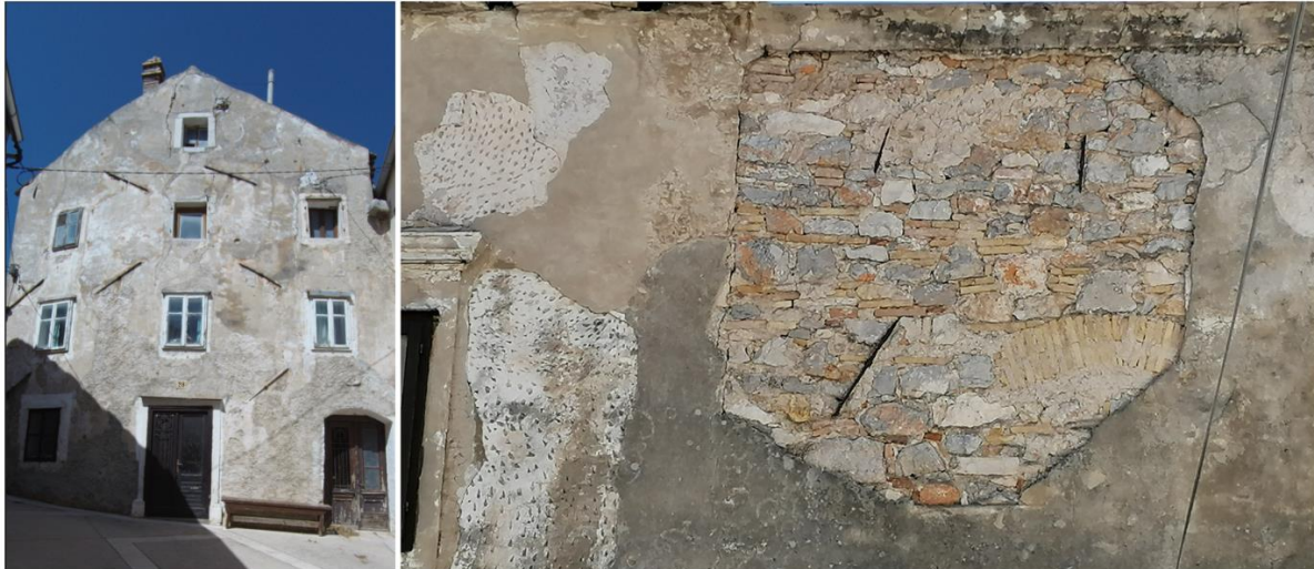
Figure 6. Tie rods visible on the facade of the building (left) and inside the section of the Wall (right)
