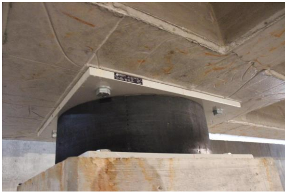
Figure 14. a) HDRB isolator SI-S 800/160
