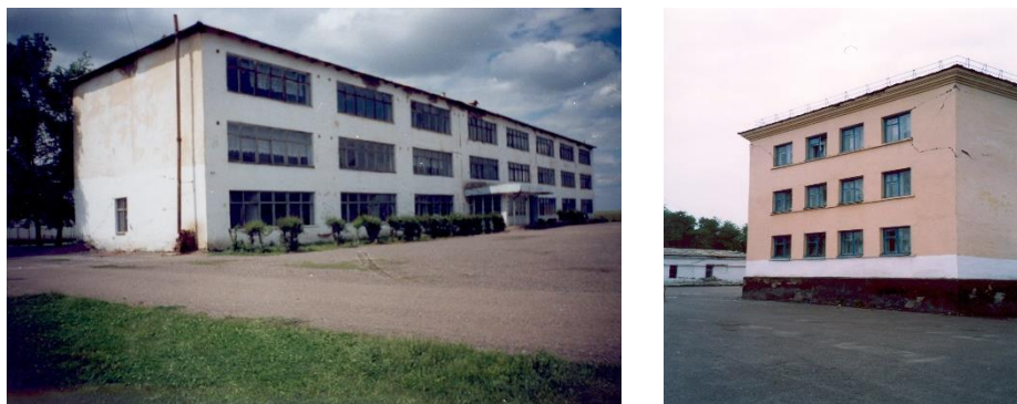
Fig. 7. General view of schools with load-bearing brick walls of complex construction
