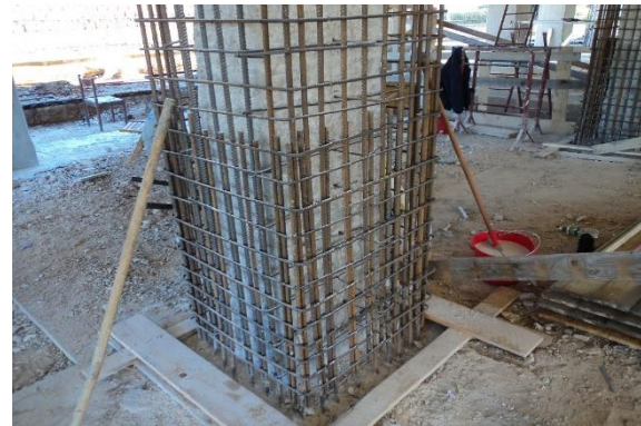
b) Increase of section and reinforcement bar in a pillar
