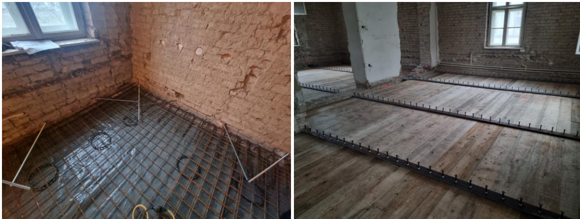
Figure 9. New stiff diaphragm
