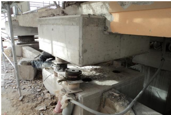
Figure 5. a) Strengthening and cutting the top of a pillar
