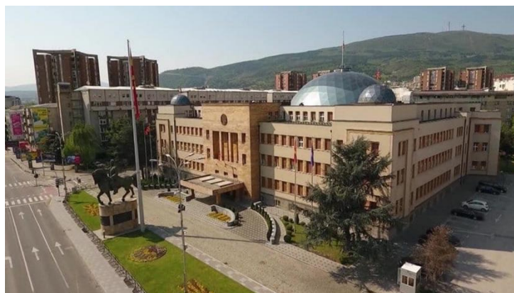
Figure 12. The Parliament building after seismic retrofitting, adaptation and building of another storey
