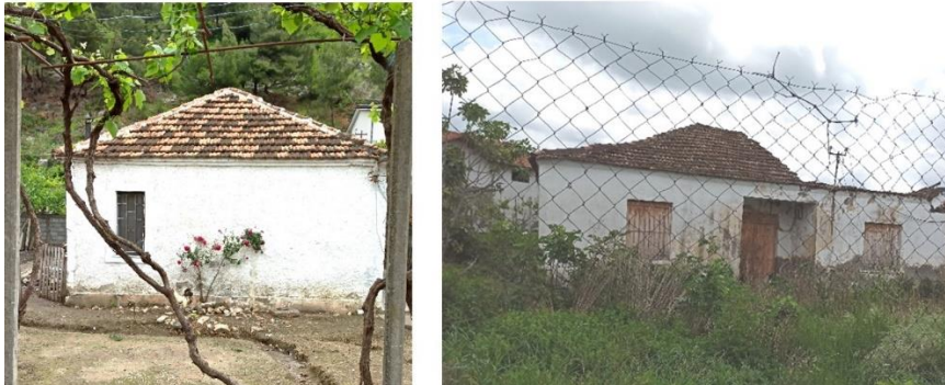
Figure 4. Examples of buildings built in the 1945-1960 period
