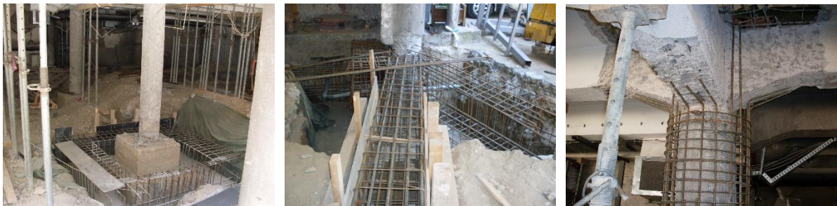
Figure 11. Strengthening of a characteristic column with a plastic hinge, unit L3
