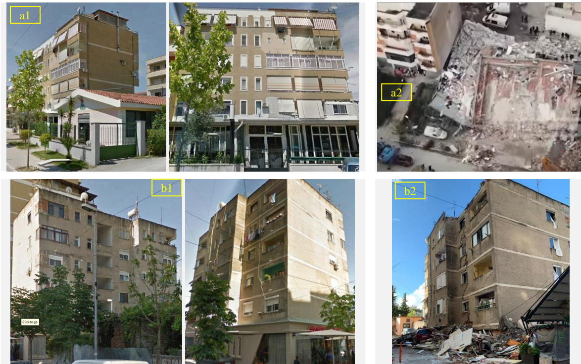
Fig. 10. Two cast-in-place M-RC 82/2 Model collapsed buildings: a-) pancake mechanism; b-) “soft story” mechanism
