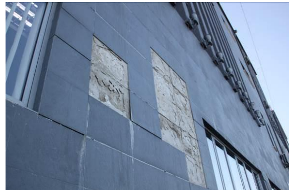
Figure 14. Cladding with ceramic tiles
