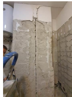
b) Interior of the sanitary unit
