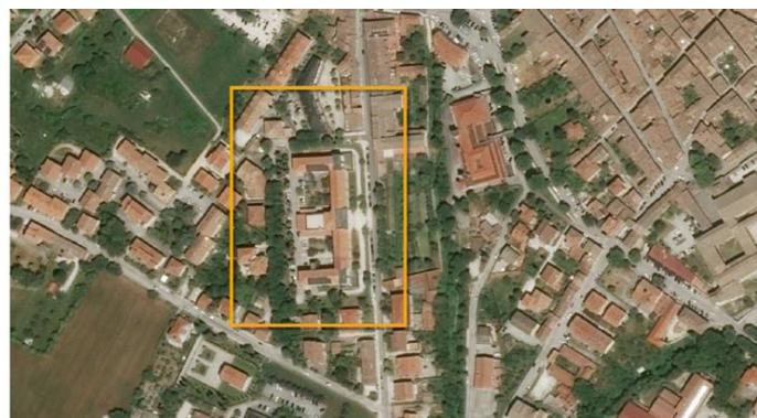
Figure 1. Identification of the building.
