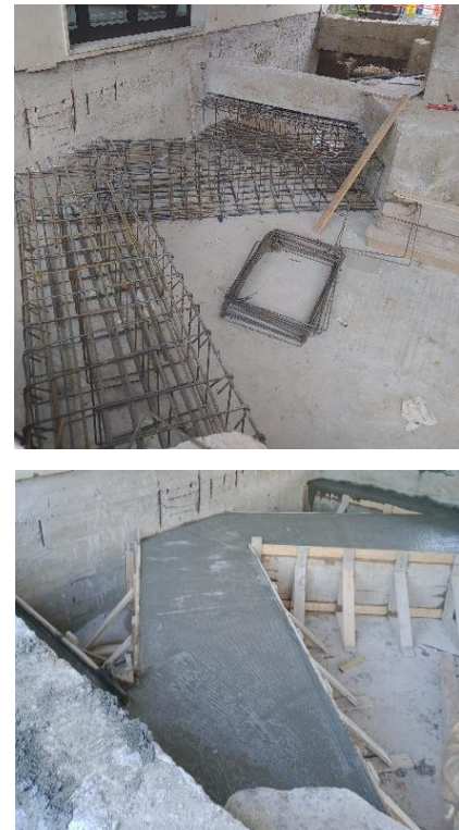
Figure 13: Detail of connecting beams realized among the foundation
