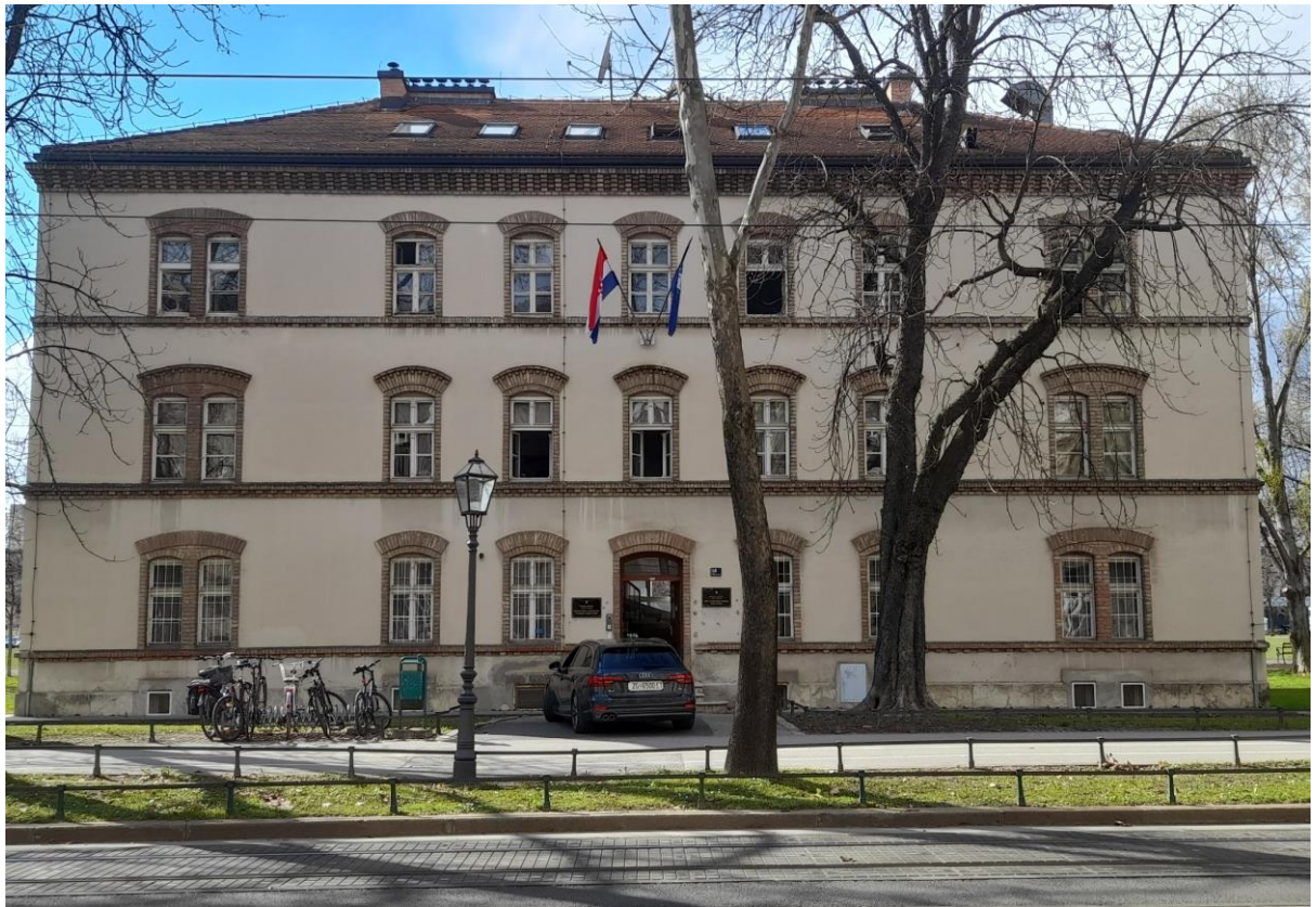
Figure 1. Case study building
