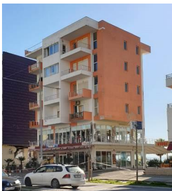
Figure 3. Non-uniform distribution of non-structural components
