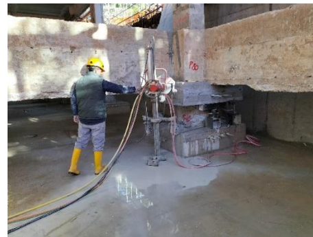
6) cutting the top of the pile with diamond wire;
