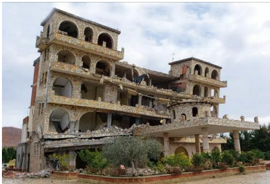
Figure 13. Cladding with natural stone
