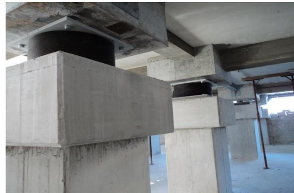
Figure 6. a, b) Level 0 with all isolators at the top of strengthened pillars
