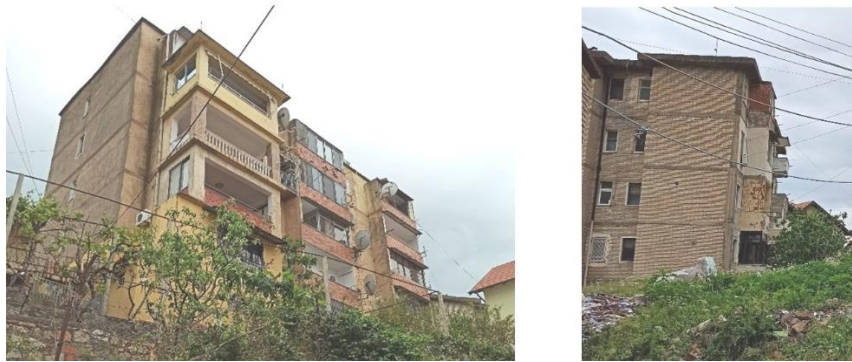
Figure 6. Examples of buildings built in the 1979-1990 period
