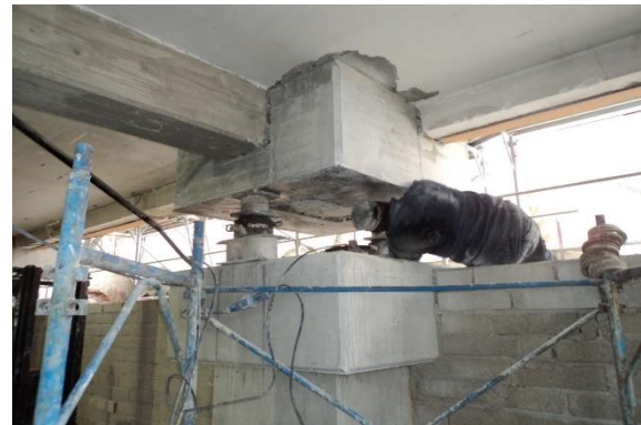
b) Control of the cutting of a pillar
