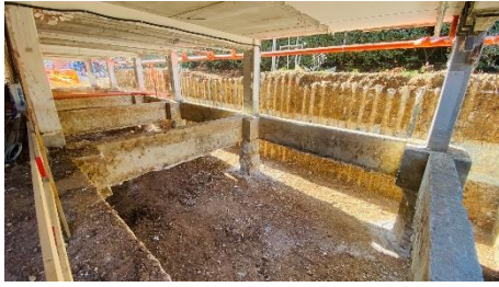
1) excavation below the existing foundation beams;
