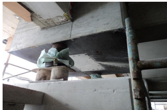
b) Cutting a pillar for isolator insertion
