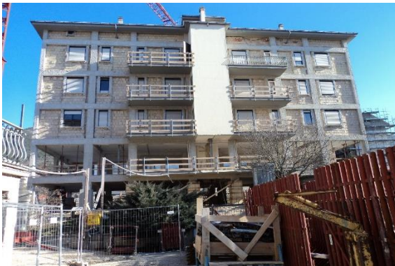
Figure 8. a) Building # 2 (six storeys)
