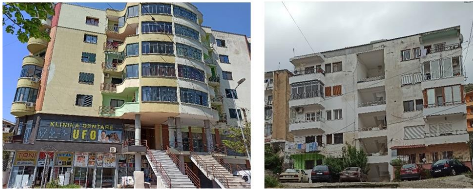
Figure 7. Examples of buildings built in the 1990-2000 period
