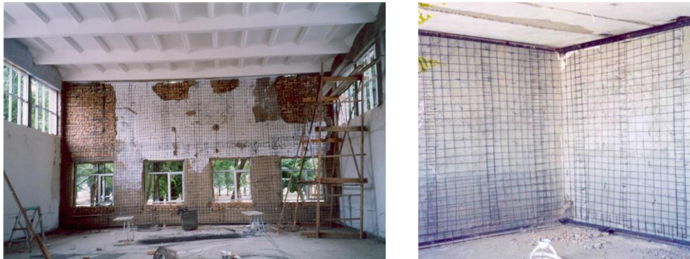
Fig. 10. Reinforcement of brick walls with reinforcement grids
