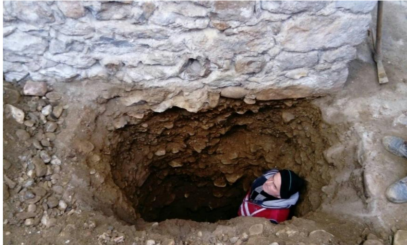
Figure 3. An exploratory borehole along the northeast corner of the tower
