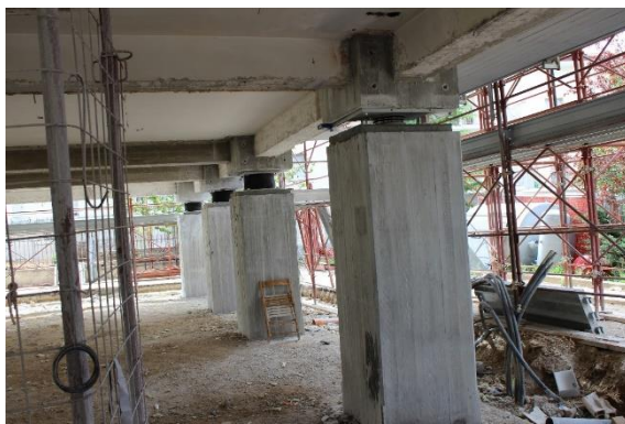
Figure 10. a) HDRB and sliding devices at top of pillar
