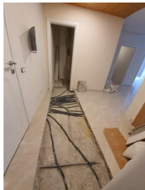
a) interior of the corridor
