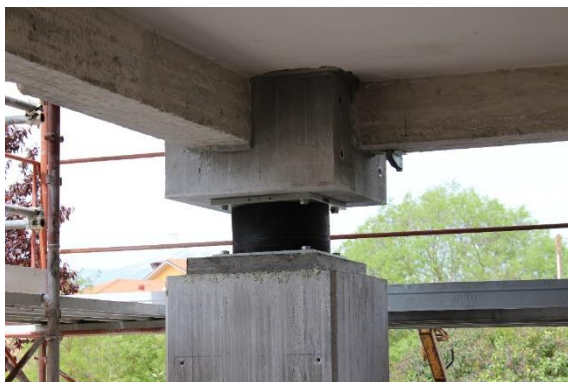
Figure 11. a) HDRB rubber isolator SI/N 450/126
