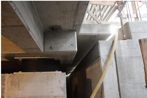
Figure 15. a) HDRB isolator with external seismic joint
