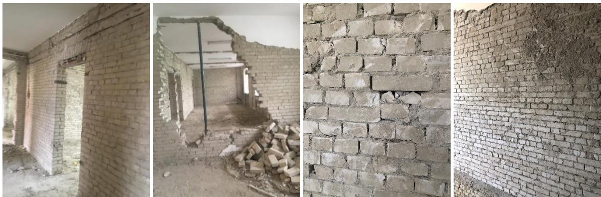
Figure 3. Wall after demolishing mortar.
