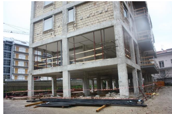
b) damage end demolition of the infills
