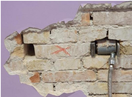
Figure 3. Masonry shear strength testing
