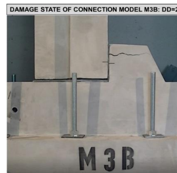
Fig. 12. Damage degree of model M3-B: Typical stage characterized by DD=2.
