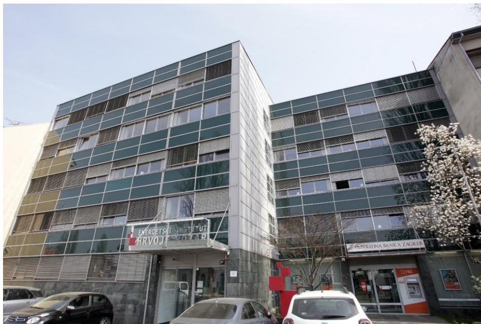
Figure 3. Front view of the case study building
