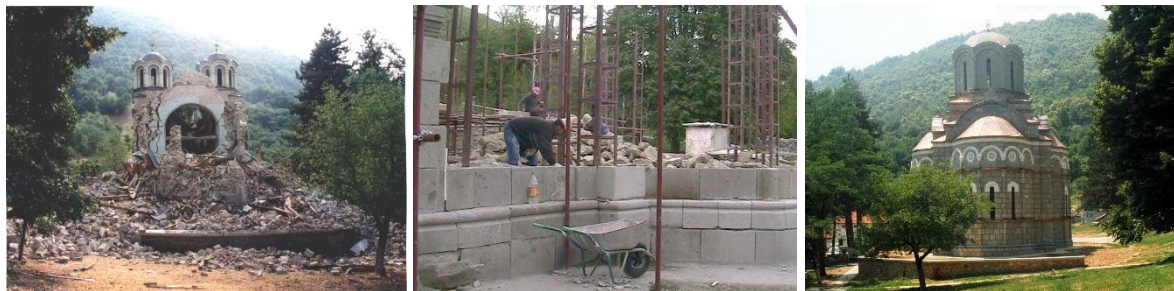
Figure 6. St. Athanasius church: after detonation, (left) during reconstruction, (middle), rebuilt church (right)
