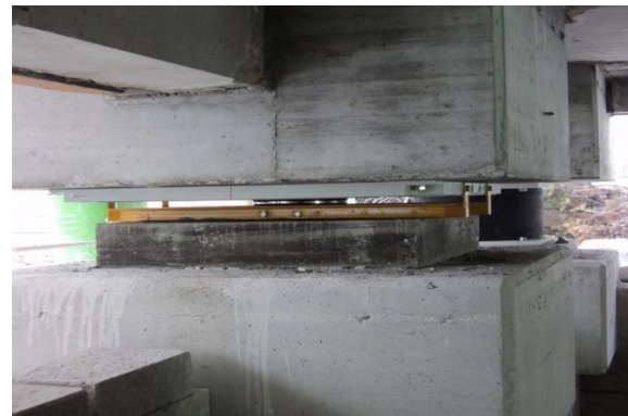
b) Insertion of a slider Vm 250/700/700
