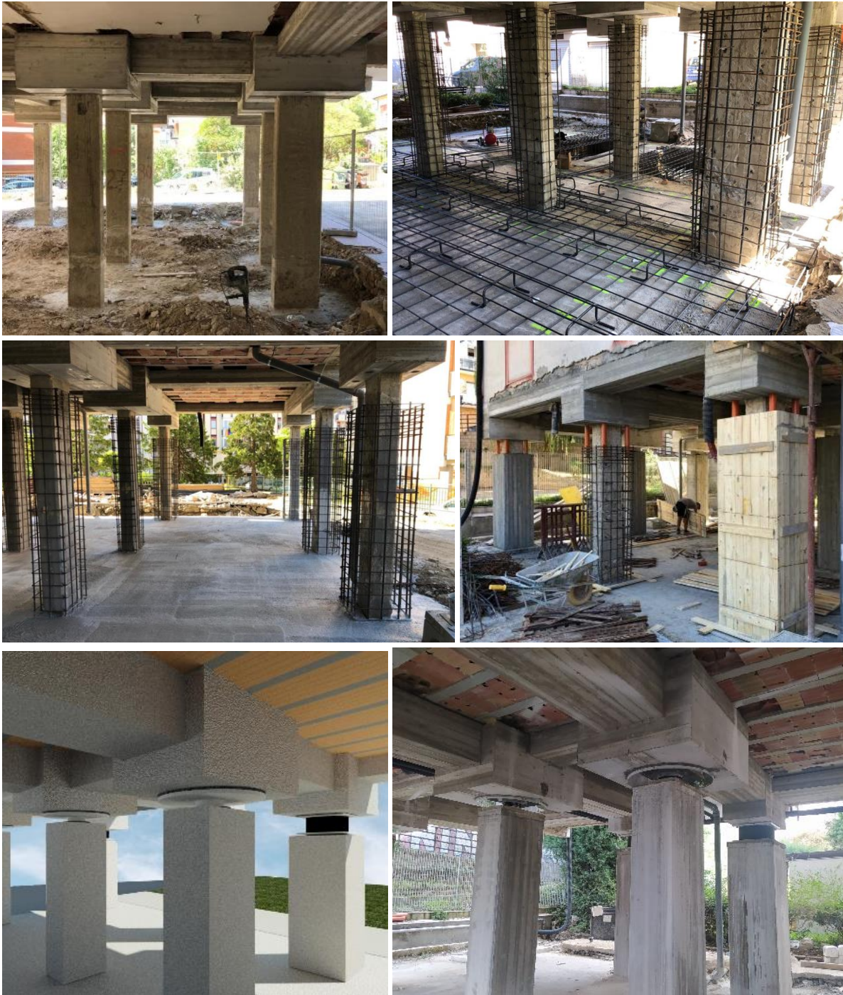
Figure 17: Details of the interventions realized
