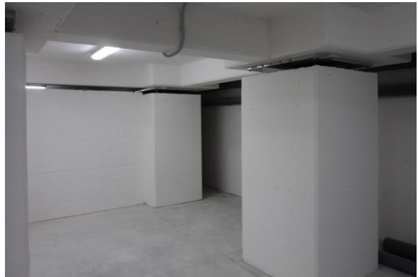
b) Horizontal joint with superstructure
