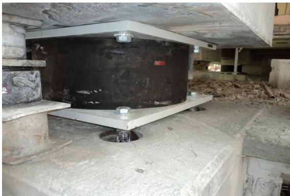
Figure 6. a) Insertion of an elastomeric HDRB SI-S 800
