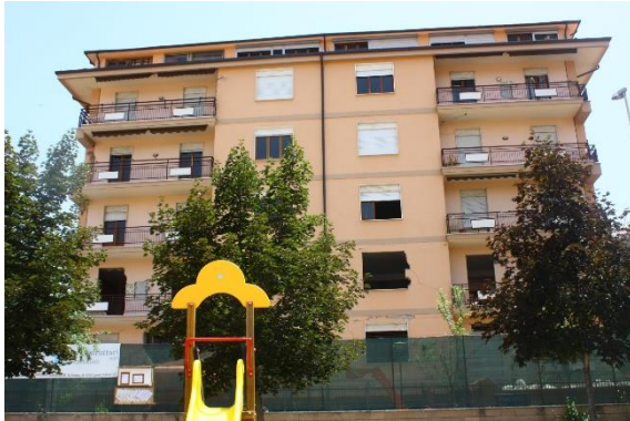
Figure 4. a) Building # 1 (seven storeys)
