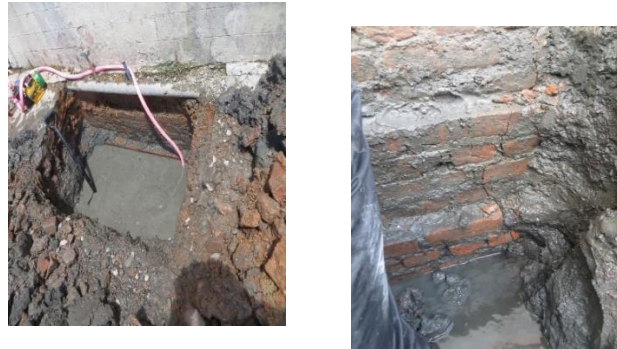
Figure 3 e) Foundation Investigation
