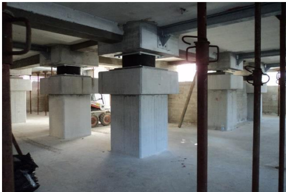
Figure 6. a, b) Level 0 with all isolators at the top of strengthened pillars
