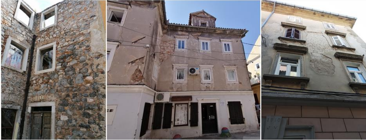
Figure 3. The facades of buildings within the historic city center of Senj
