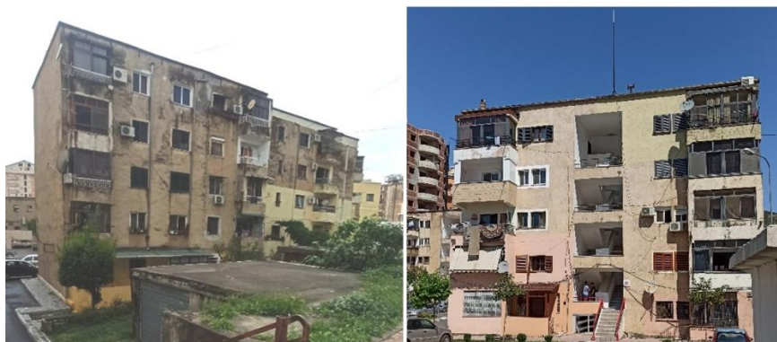
Figure 5. Examples of buildings built in the 1960-1979 period
