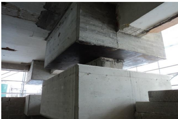
Figure 5. a) Strengthening of a pillar
