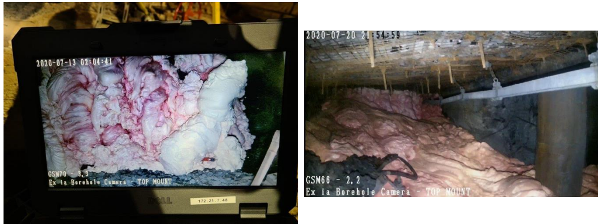
Figure 2. Tunnel seal – Rocsil foam
