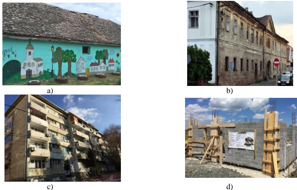
Figure 2. Examples of masonry building typologies from Serbia: a) M1- a single-family building in Irig (Vojvodina); b) M2 – an early 20 th century URM building in Zemun; c) M3-M – an apartment building in Belgrade; d) M4- a single-family house under construction, Zlatibor.
