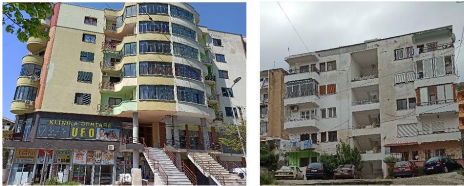
Figure 7. Examples of buildings built in the 1990-2000 period
