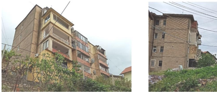
Figure 6. Examples of buildings built in the 1979-1990 period
