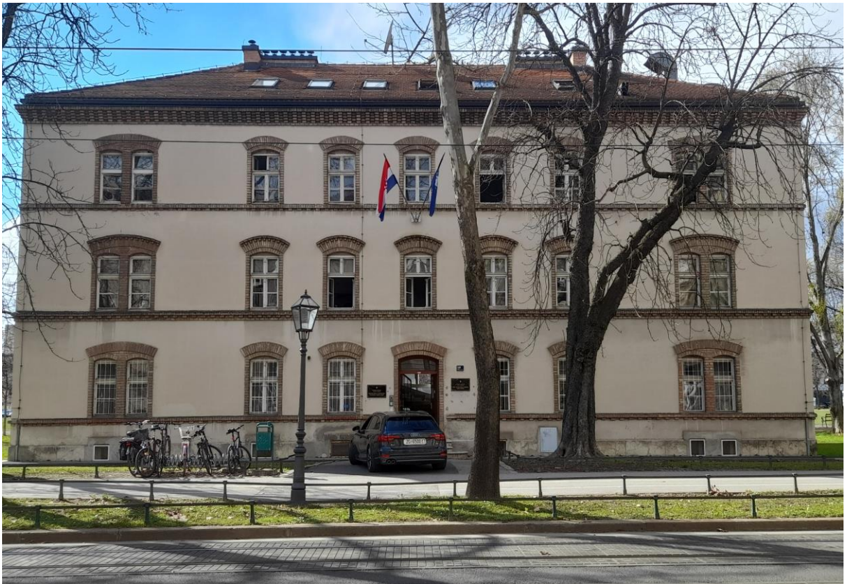
Figure 1. Case study building
