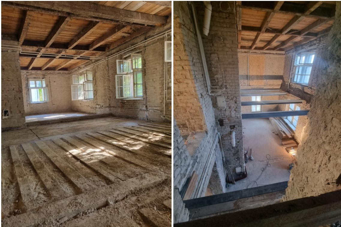
Figure 8. Plaster removal and preparations for strengthening
