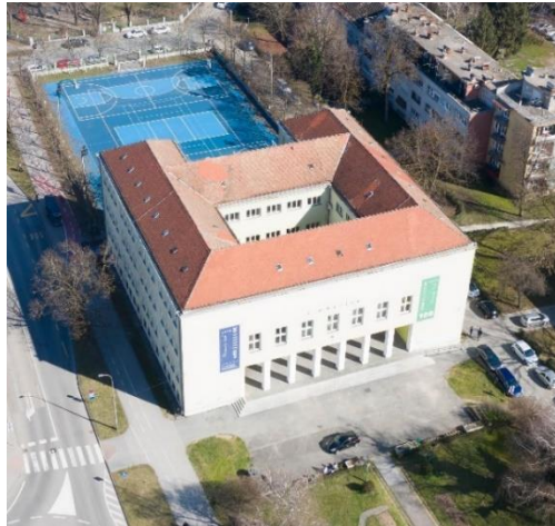
Figure 1. Sisak highschool building
