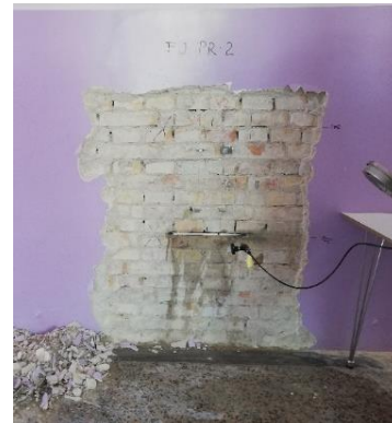
Figure 4. The determination of the existing compressive stress in the masonry
