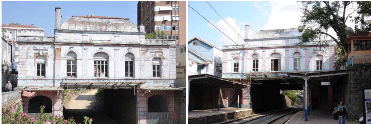
Figure 8. Recent Photographs of the Station Before Strengthening
