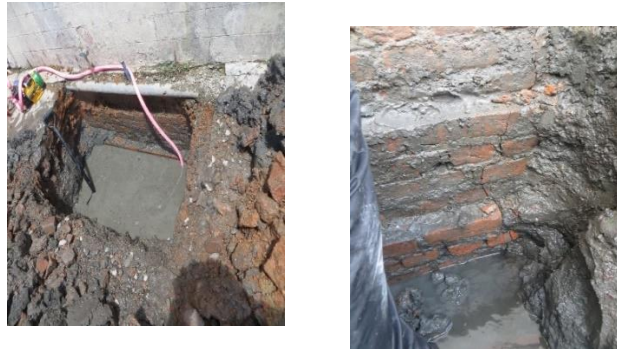
Figure 3 e) Foundation Investigation
