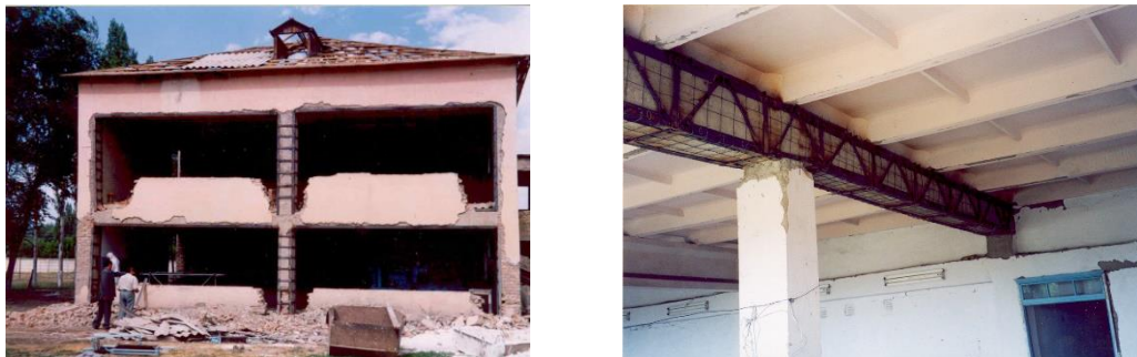
Fig. 11. Reinforcement of columns and beams with steel clips
