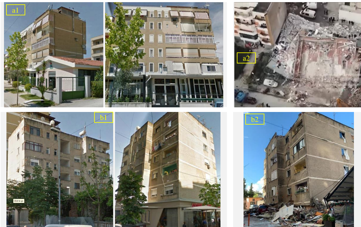
Fig. 10. Two cast-in-place M-RC 82/2 Model collapsed buildings: a-) pancake mechanism; b-) “soft story” mechanism
