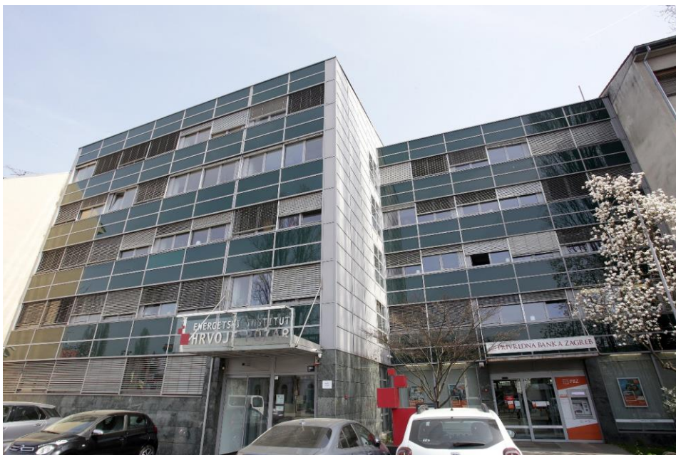
Figure 3. Front view of the case study building
