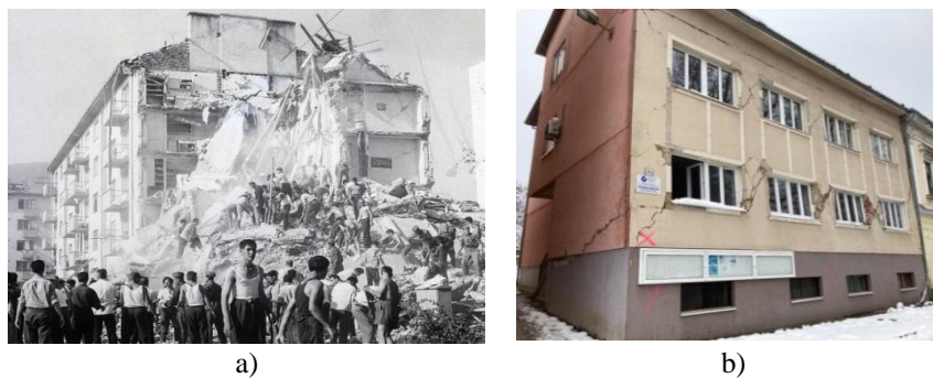
Figure 2. Performance of URM multi-family residential buildings in past earthquakes in the region: a) a collapsed building due to the 1963 Skopje earthquake (credit: Z. Milutinović) and b) a damaged building due to the 2020 Petrinja earthquake (credit: SUZI-SAE).
