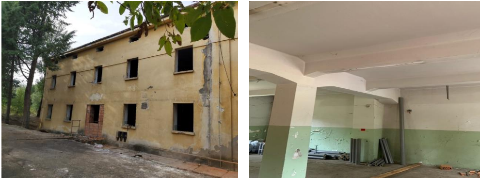
Figure 1. Façade of the building and building interior
