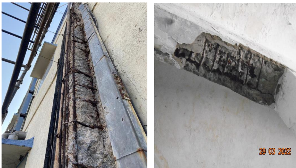
Figure 4: Existing condition of Columns and Beams
