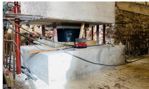
d) Installation of isolator
