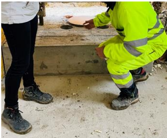
c) Installation of flat jack
