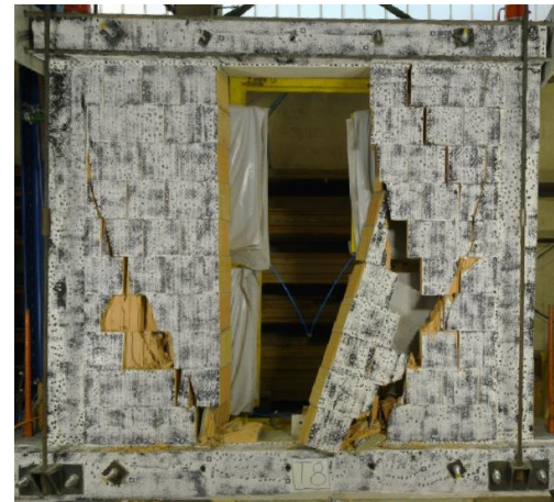
Figure 8. Collapse of masonry infill at 1.6 % of in-plane drift
