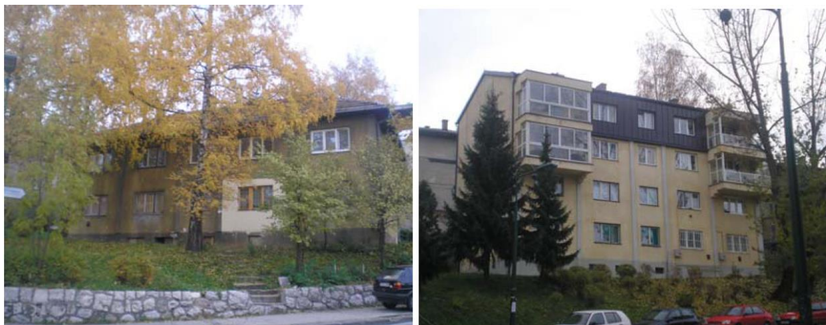
Figure 1. Masonry building before reconstruction (left), after reconstruction (right).
