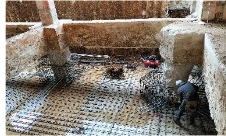
2) placing reinforcement for the new structure (plinths and foundation slab);
