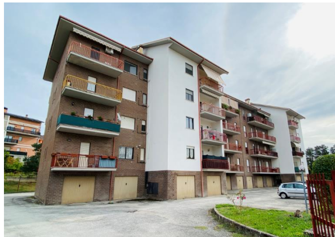
Figure 7. The building in via Di Vincenzo 23.
