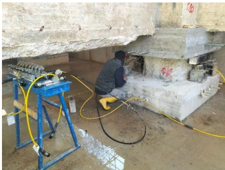
5) placing of hydraulic jacks and displacement transducers;
