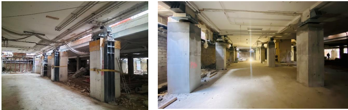
Figure 5. Crefel Building: two phases of the installation of the isolators.
