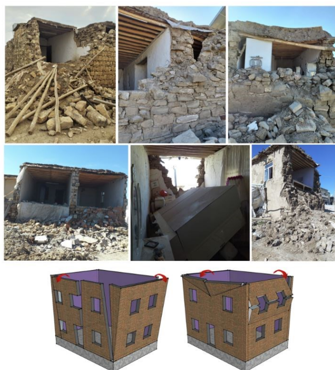
Figure 1. OOP failure mechanisms observed in URM structures [8].
