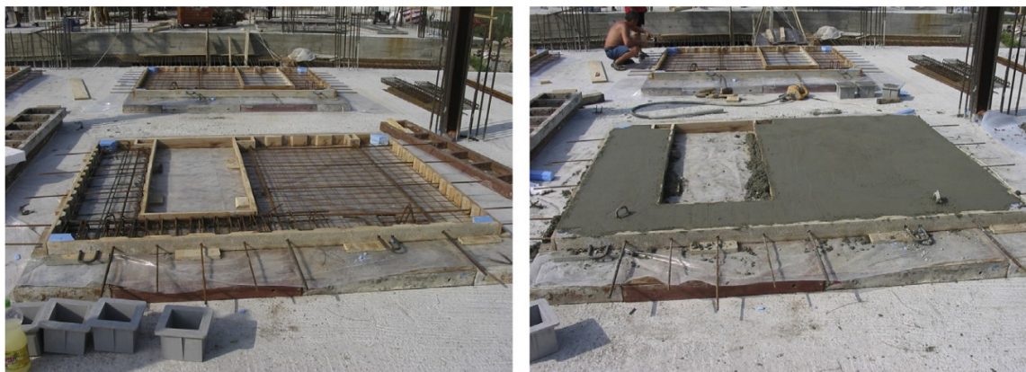
Figure 2. Manufacturing process for plain wall panel [18]
