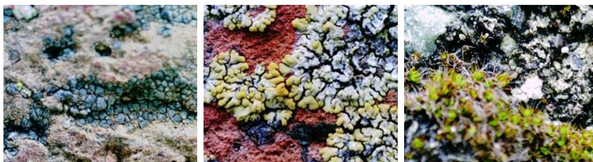
Figure 3.4 Different types of lichens present on the facades of the church (magnification 40x)
