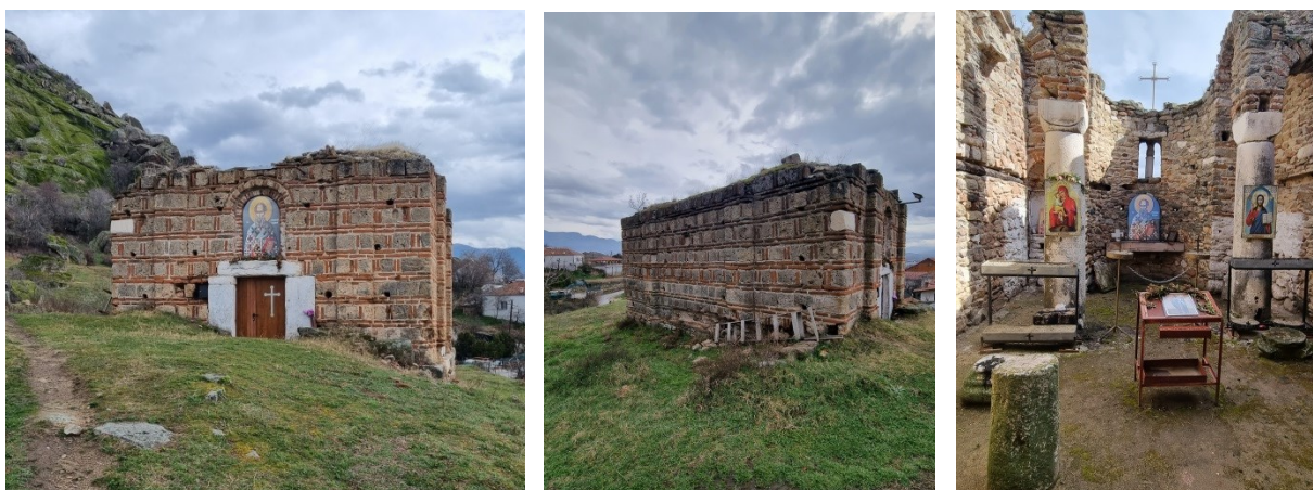
Fig. 3.8 Exterior and interior of the St. Atanasius church in Varosh, Prilep
