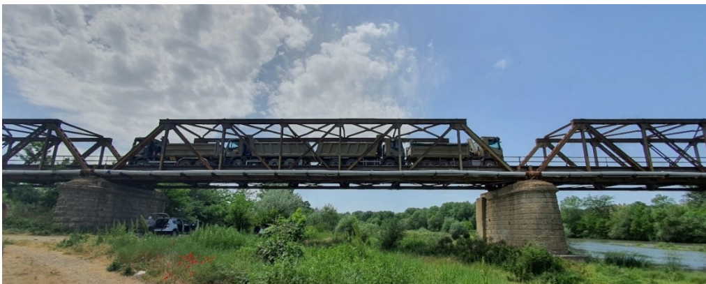
Figure 9. Photo of static loading of section 2
