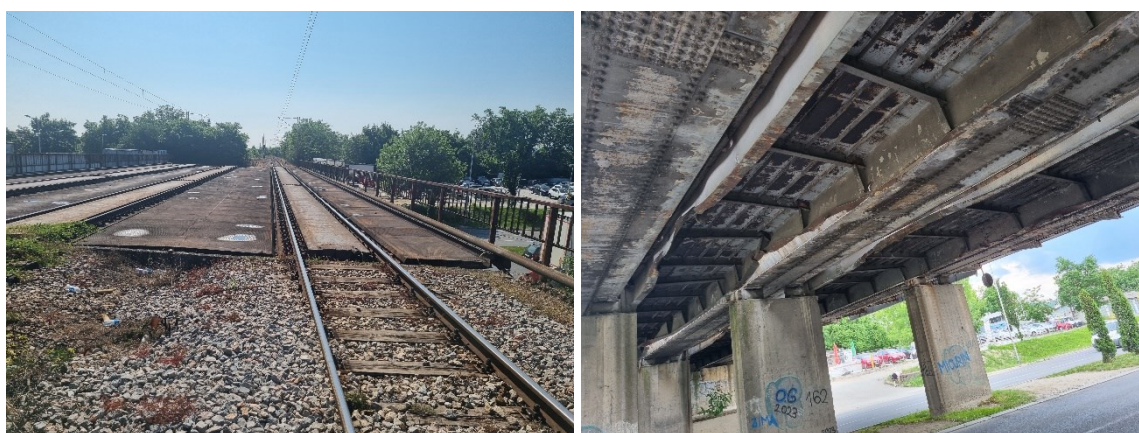
Figure 2. View above (left) and below (right) the simply supported steel girder underpass.
