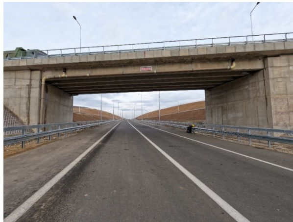
Figure 8. View of the prestressed reinforced concrete overpass with the installed radar for measurement.
