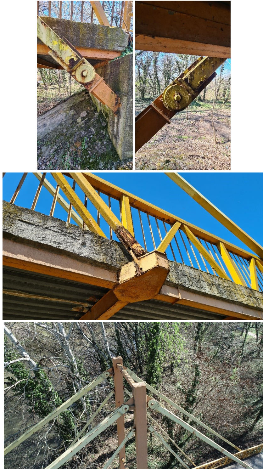
Figure 6. Corrosion detection following visual and UAV inspection.
