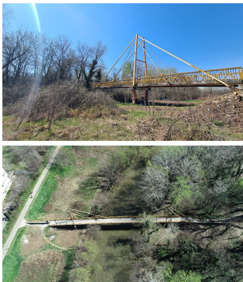
Figure 5. Side view (top) and view from aerial perspective (bottom) of the cable-stayed pedestrian steel bridge.
