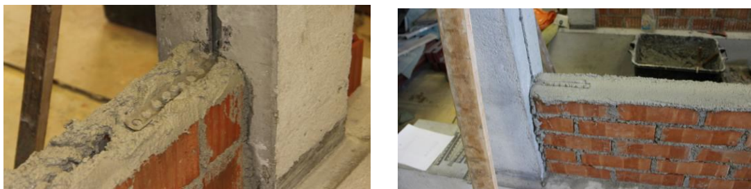
Figure 6. a and b, Positioning of wall tie anchors: a: clay blocks and b: clay brick masonry
