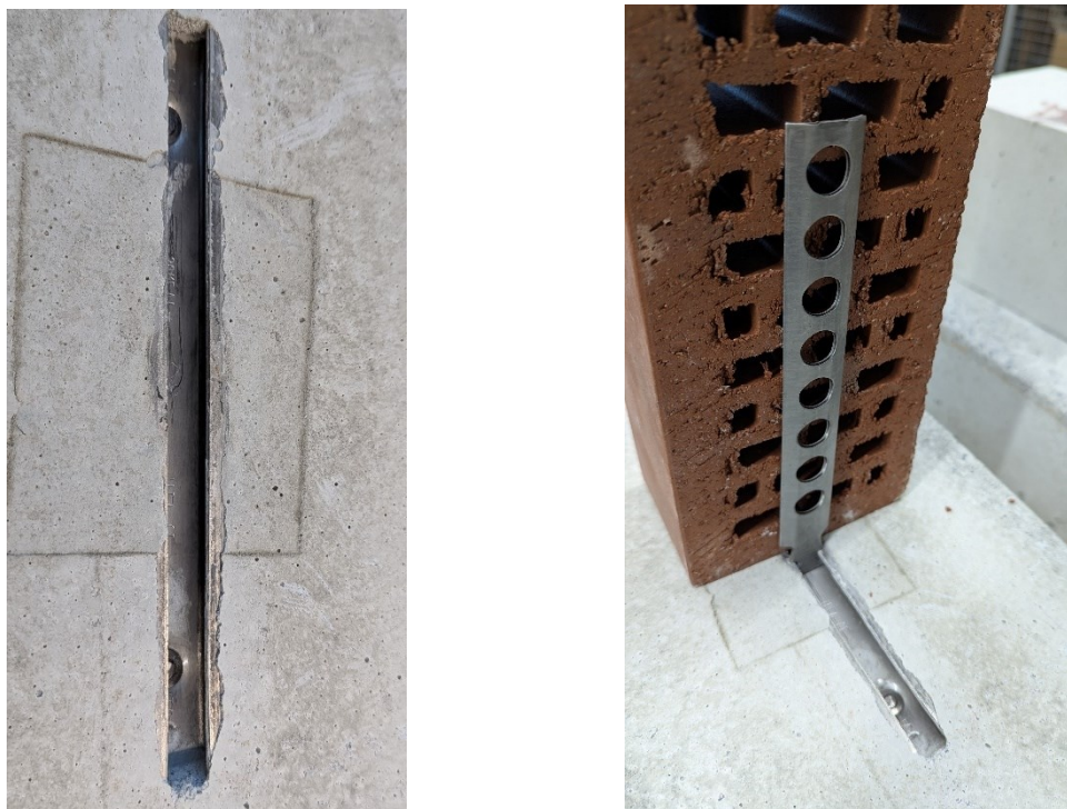
Figure 1. a) cast-in anchor channel; b) flat anchor interlocking with the channel.
