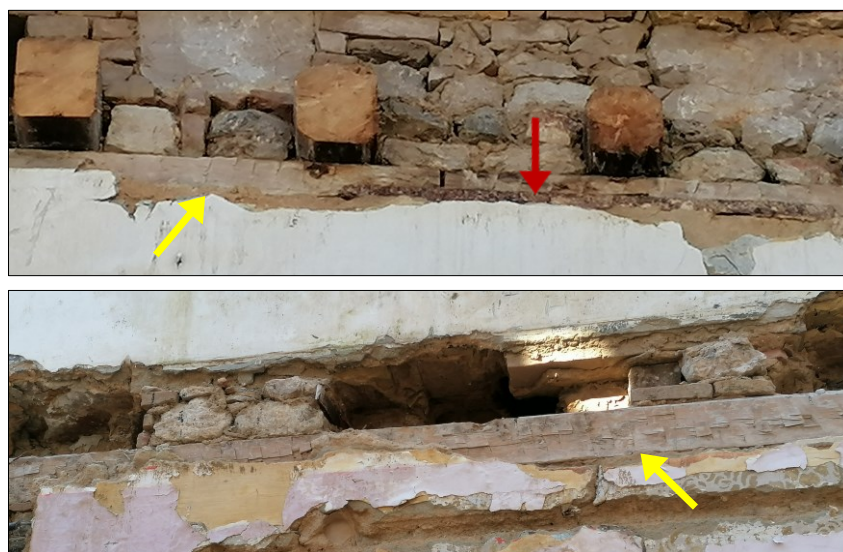
Figure 5. Timber ring beams at the floor levels.
