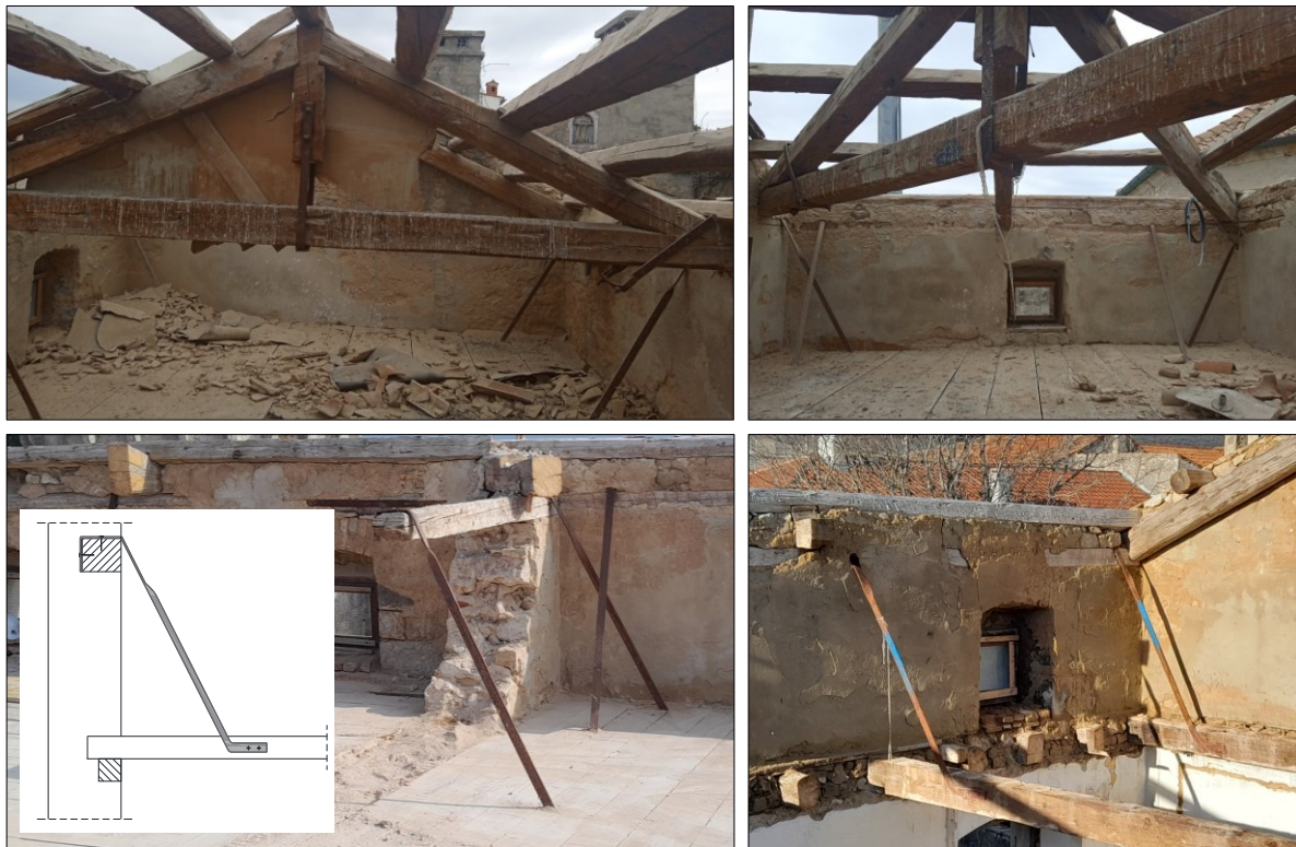
Figure 8. a) Diagonal wall-to-floor iron ties.
