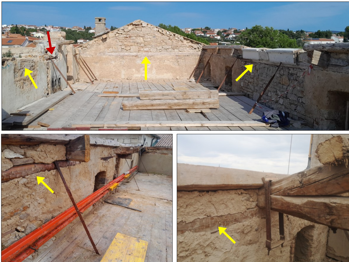
Figure 4. Timber ring beams at the roof level.
