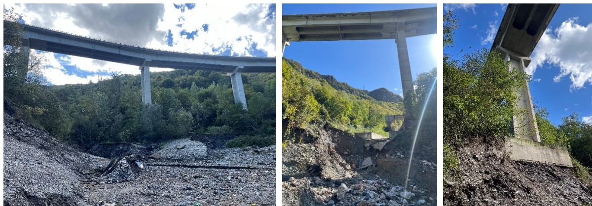
Figure 6. Photographs of key structural elements of the inspected bridges and the eroded terrain in the area of pier foundations
