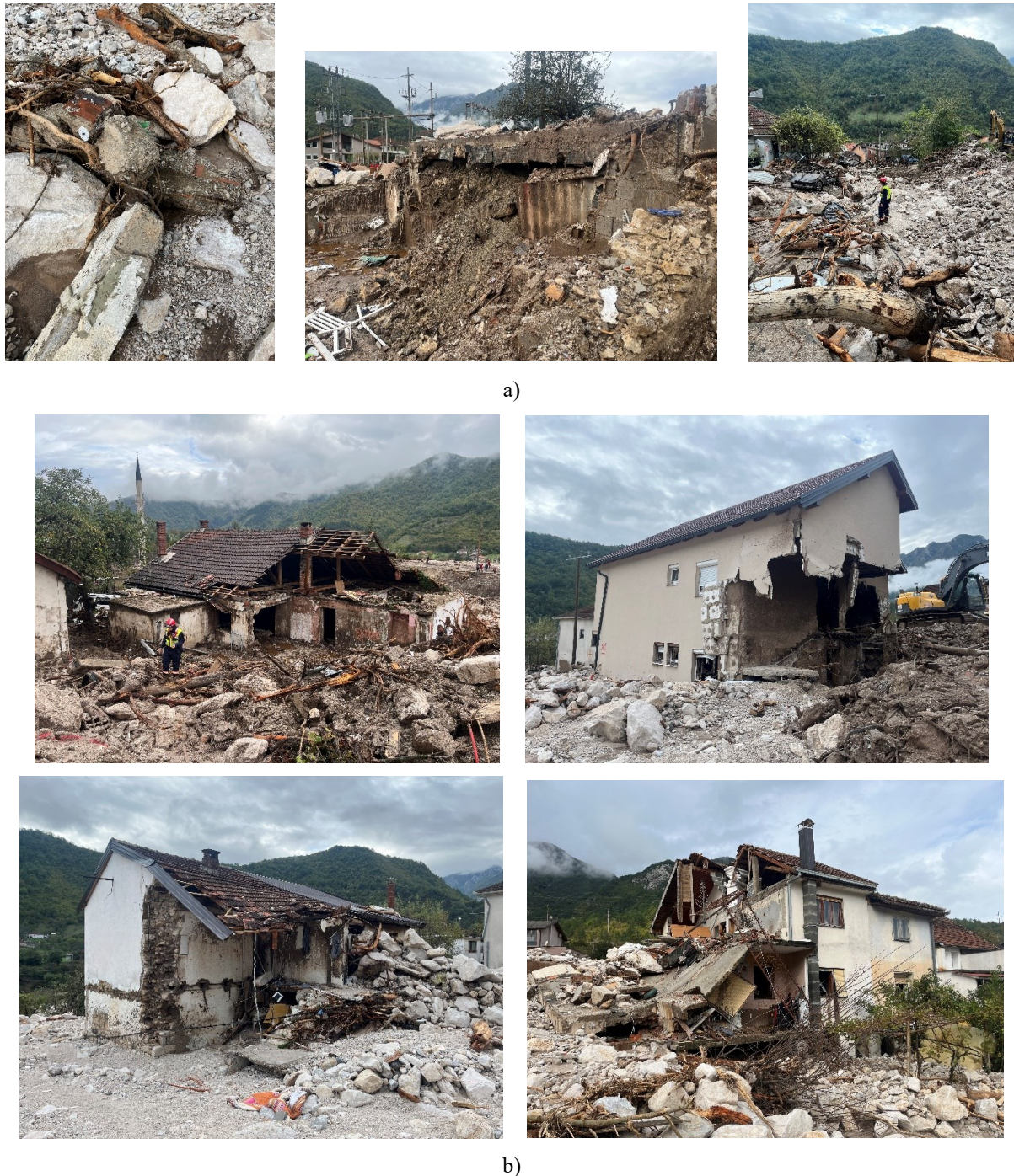
Figure 2. INSARAG collapse types observed in Donja Jablanica; a) debris heaps, b) overhanging elements
