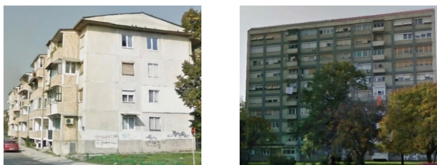
Figure 10. Prefabricated reinforced concrete structures of the “Karposh” system, Skopje (RC3)
