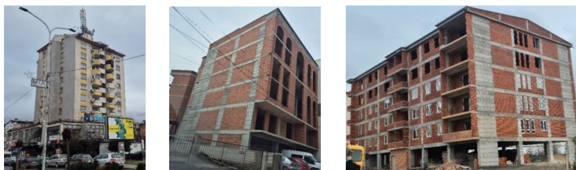
Figure 9. Reinforced concrete frames with shear walls, Gostivar (RC2).
