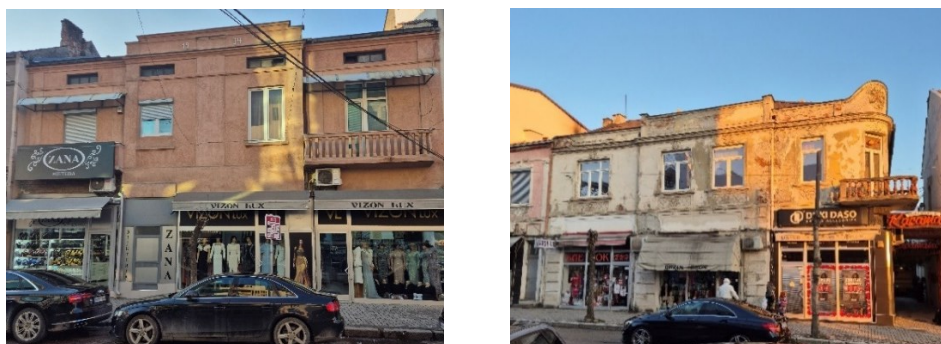
Figure 5. Unreinforced masonry with solid firebricks and wooden flexible floor, Gostivar (URM2).
