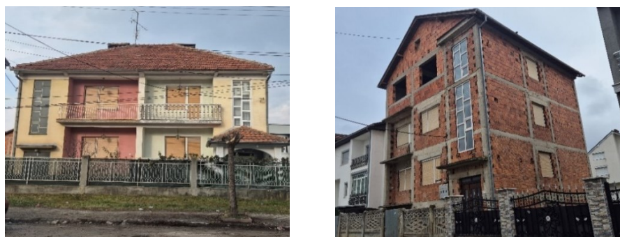
Figure 7. Confined masonry with solid bricks or hollow blocks, Gostivar (CM).
