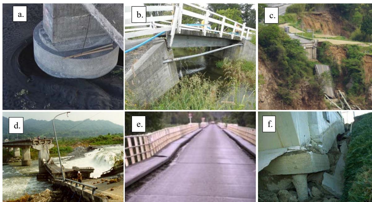
Figure 2. Examples of soil damage: a. liquefaction [25]; b. embankment fracture [26]; c. landslide [27]; d. bridge collapse due to fault 7 m upthrust [28]; e. column settlements causing superstructure deflections [26]; f. heavy damage to foundation piles [29]
