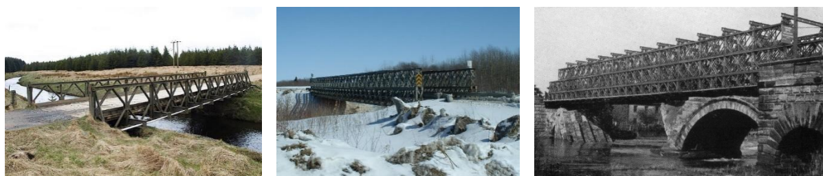
Figure 3. Bailey Bridges: single-truss single-story (SS), double-truss double-story (DD) and triple-truss triple-story (TT)
