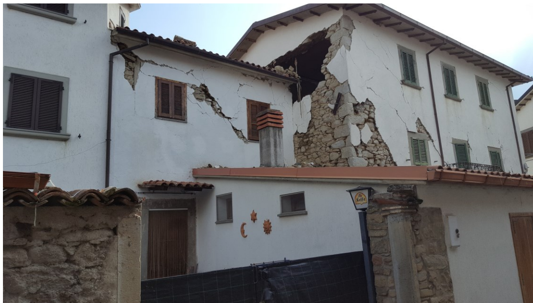
Figure 1. Local mechanism and in-plane damage in existing aggregates in Amatrice, Italy, after the 2016 Central Italy earthquake (Photo: A. Penna/G. Guerrini).
