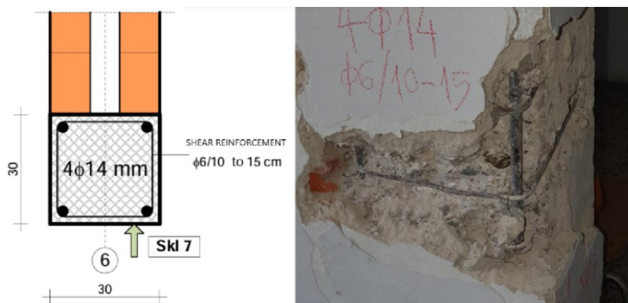
Figure 3. Reinforcement in the column [4]
