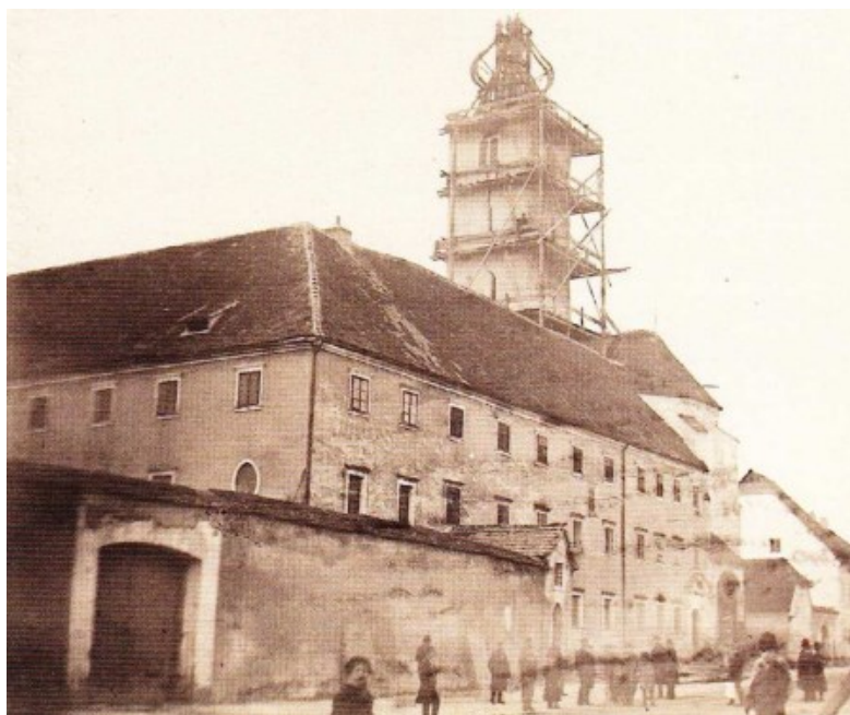
Figure 3. Removing the cap from the belfry of the Church of St. Francis of Assisi in Zagreb after the earthquake of 1880. [2]
