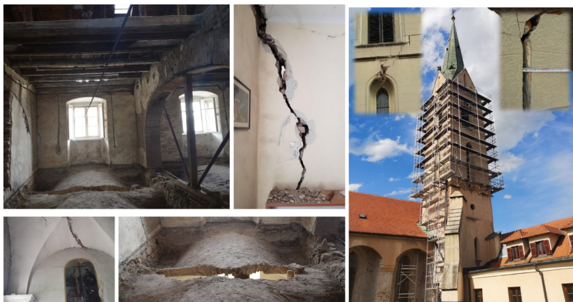
Figure 5. Photos of some damage to the structural parts of the Franciscan complex [1, 4]
