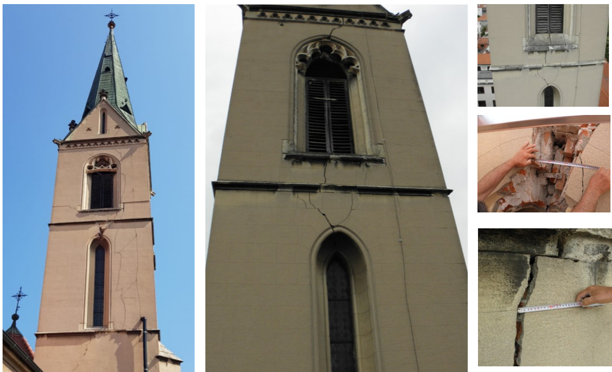
Figure 16. Belfry damage [5, 1]
