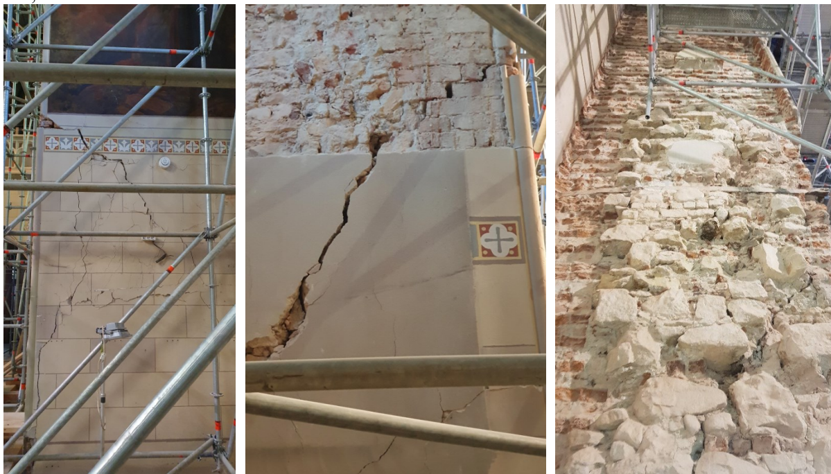
Figure 7. Damage to the church's buttresses [1, 5, 4]
