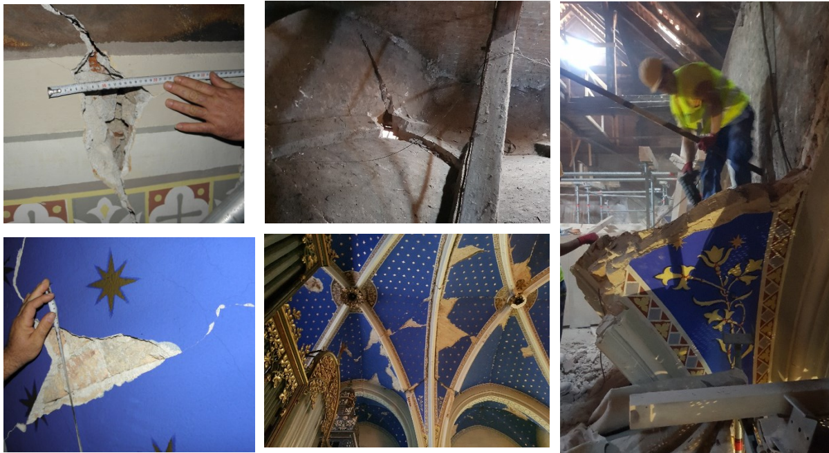
Figure 10. Damage to the church vaults [4, 5]
