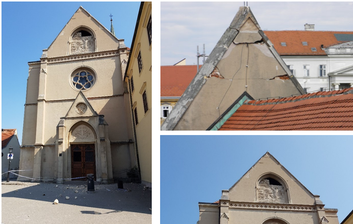
Figure 13. Damage to church walls [1, 5]
