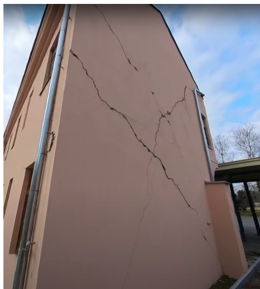
Figure 2. Damage to a building in Sisak that is about to be demolished
