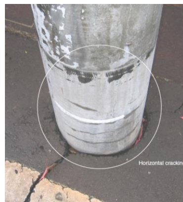
Figure 8. Horizontal cracking near the base of the poles [3]
