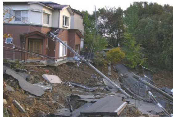
Figure 2. Utility poles damaged by landslide [3]
